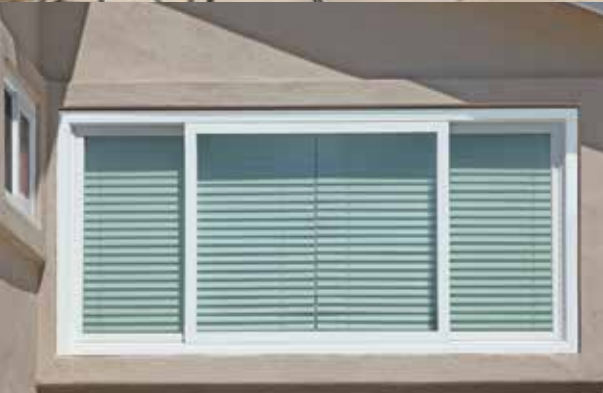
Double slider with Z-bar on stucco
